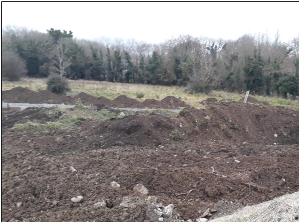
Figure 13: The loads of material (soil, stone, etc.) ready to be rolled to level the site during the infill works (image provided by the defendant David O'Toole).
